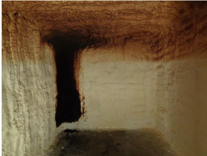
Photo No. 7 Post-test
